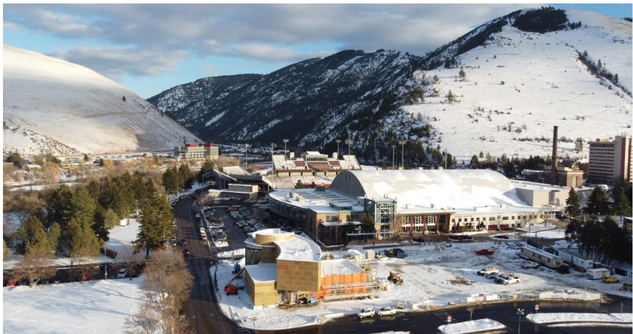
The new MMAC building taking shape along Campus Drive.
